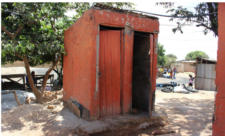
Image: Pit latrine in Chazanga, Lusaka.
